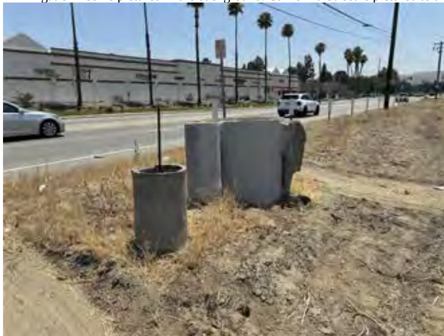
Photo 8: View of the concrete irrigation riser located along the eastern boundary of the subject site.
