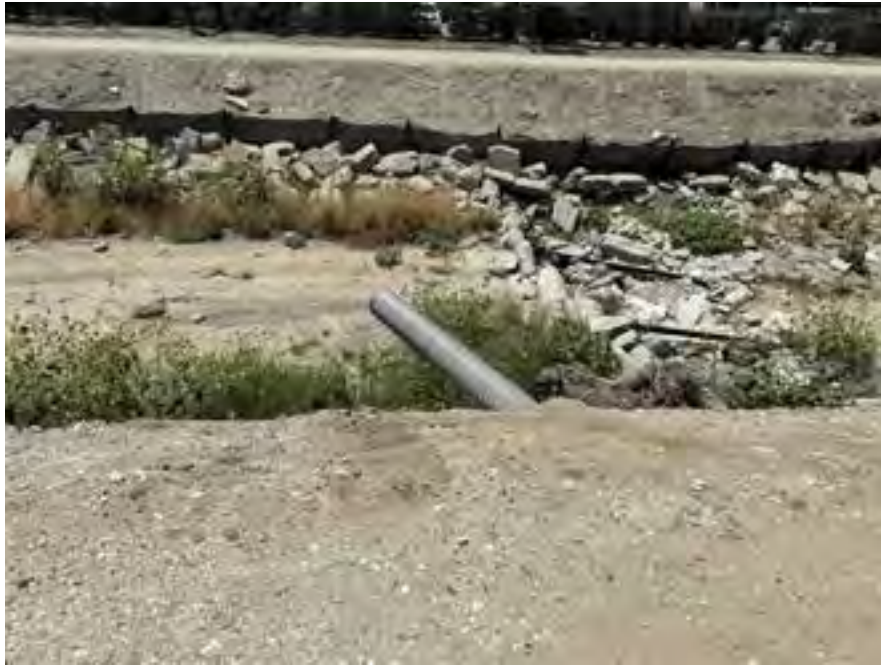
Photo 13: Western-facing view of the pipe associated with the western storm drain.
