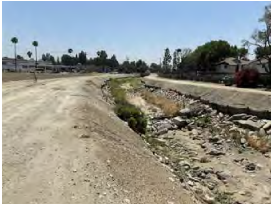
Photo 14: Southern-facing view of the canal located adjacent to the west of the subject site.
