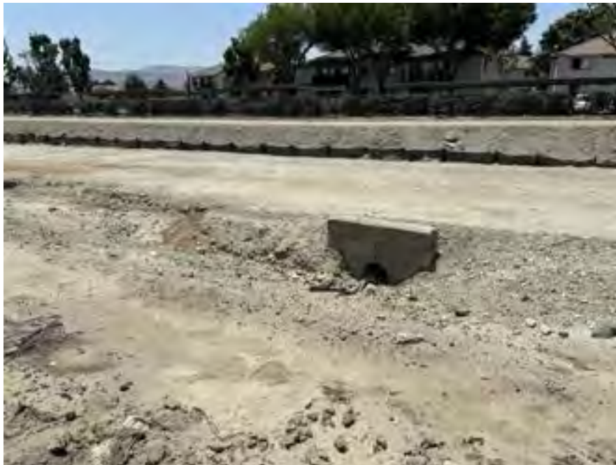
Photo 12: View of the storm drain located along the western boundary of the subject site.
