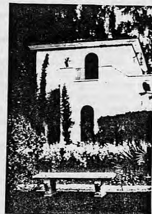
A CORNER OF THE GARAGE SHOWING THE STAIRS LEADING TO THE MAIDS' ROOMS
