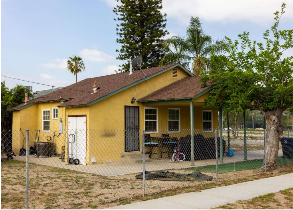
Close-up Northeast Elevation
