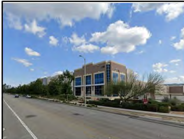
PHOTO 3: View looking south of the project site at an industrial building along West Lugonia Avenue.
