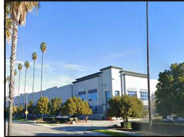
PHOTO 2: View looking east of the project site at an industrial building along California Street.
