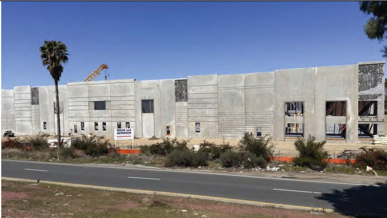
KOP 5: Existing conditions view to the northwest from Interstate 10, 34.066724, -117.226832
