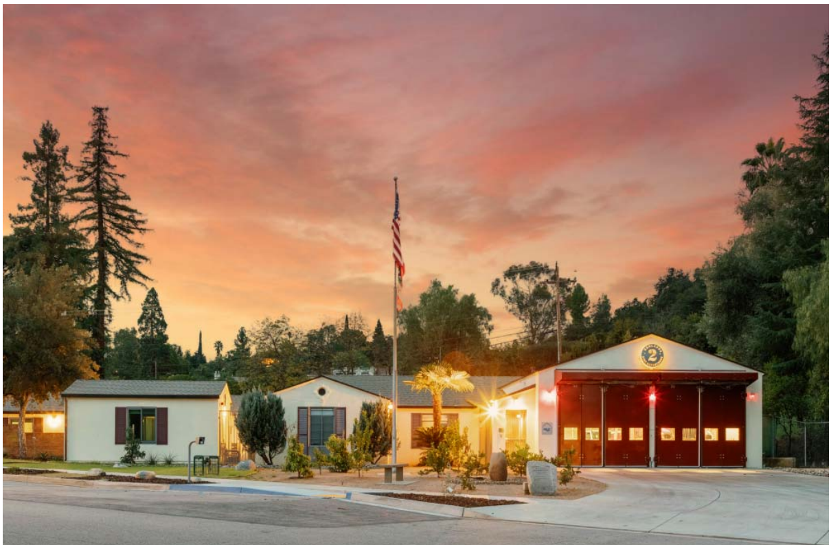
Final Completed Construction
