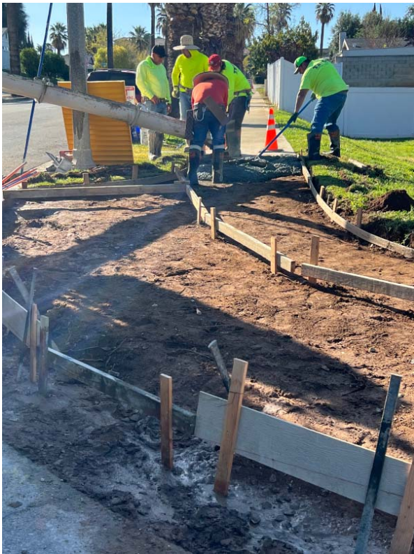
Concrete forms placed at Cambon Court
