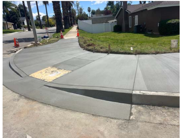
Newly installed ADA Ramp at Cambon Court
