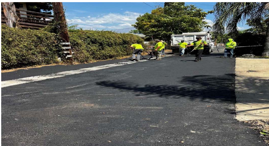
Paving work from Division Street to Chapel Street
