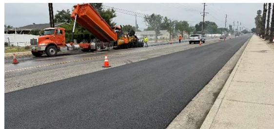
Crew performing overlay operations on San Bernardino Ave near Church St.
