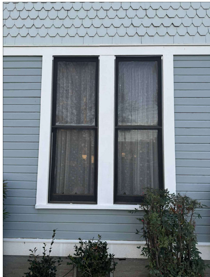
EXISTING MAIN RESIDENCE WINDOW TRIM
