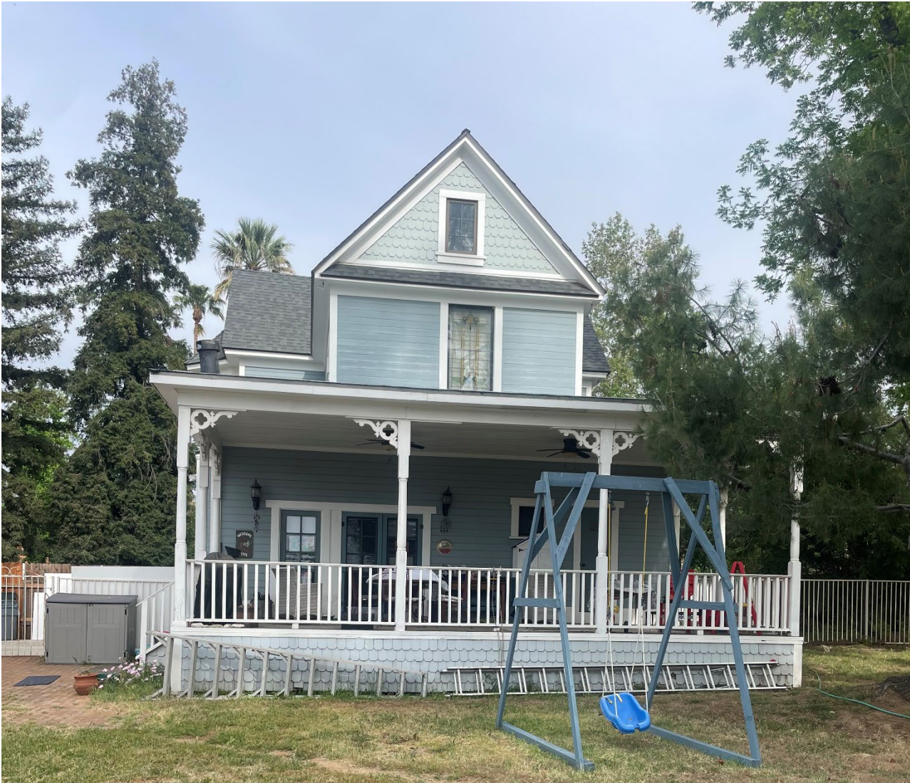
REAR ELEVATION (WEST SIDE)
