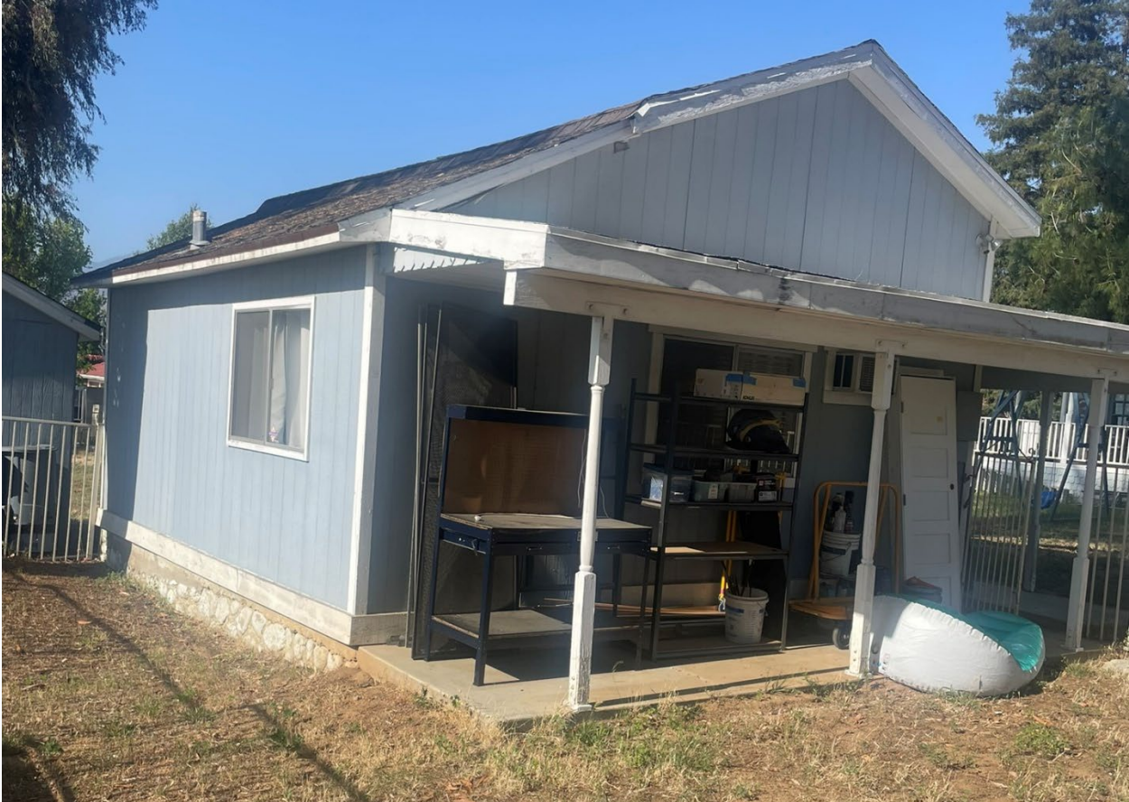
CARRIAGE HOUSE (SOUTH & WEST SIDE)
