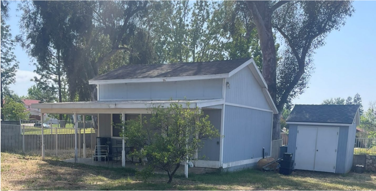
CARRIAGE HOUSE (EAST AND NORTH SIDE)
