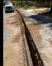
Installing an 8 Inch DIP pipe at Sunset Hills
