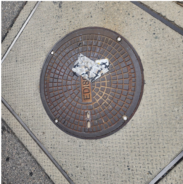
14. Edison Vault on Tennessee Street
