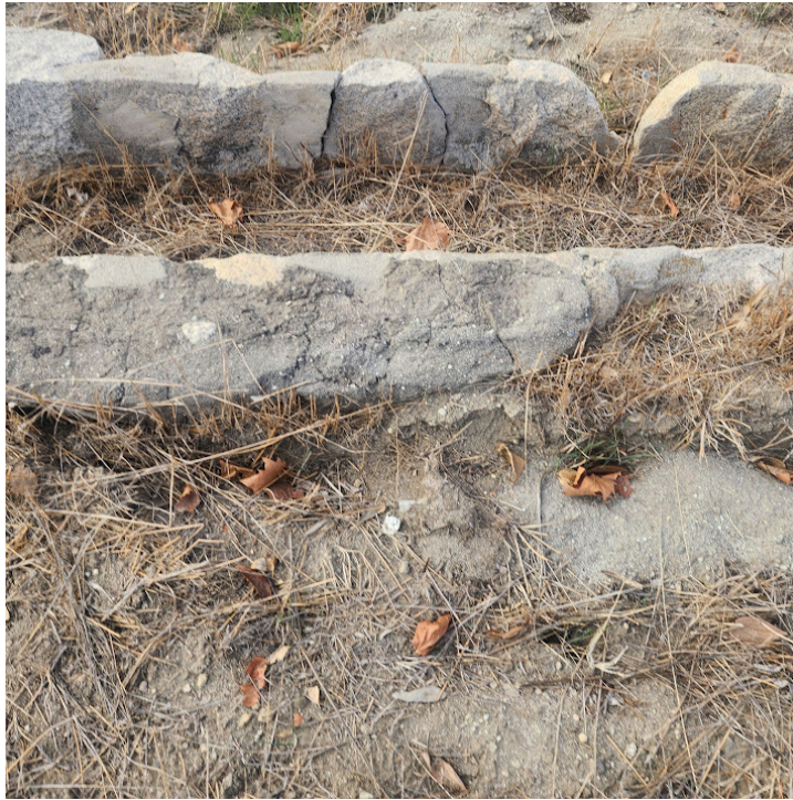
13. Former Drainage Channel
