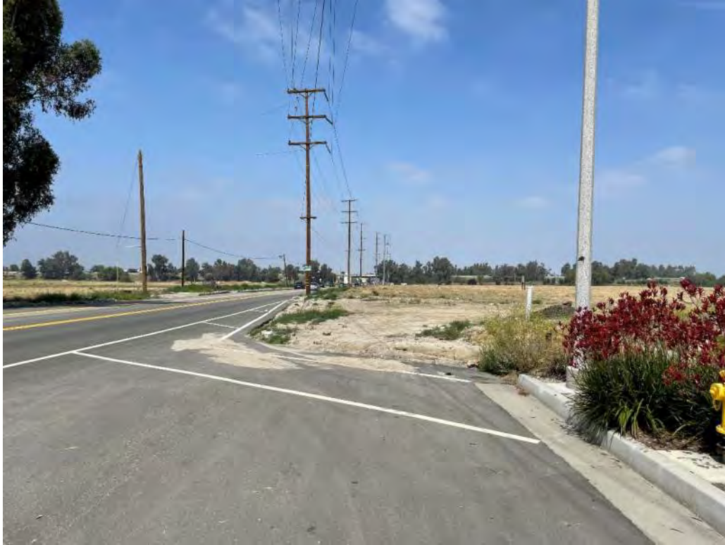
Photo 4: At southeast corner of project site on San Bernardino Avenue looking west along south project boundary.
