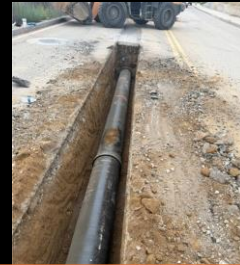
Installing 16-Inch DIP at Reservoir Rd
