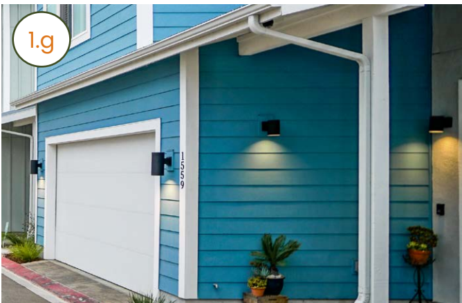
Light fixtures align with architectural theme
