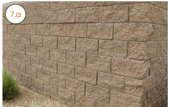
Block wall enhanced with decorative finish
