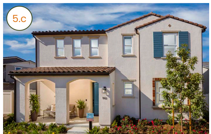
A clearly defined primary entry to the home through use of a front porch
