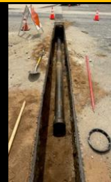
Installed 8" DIP on Opal Way
